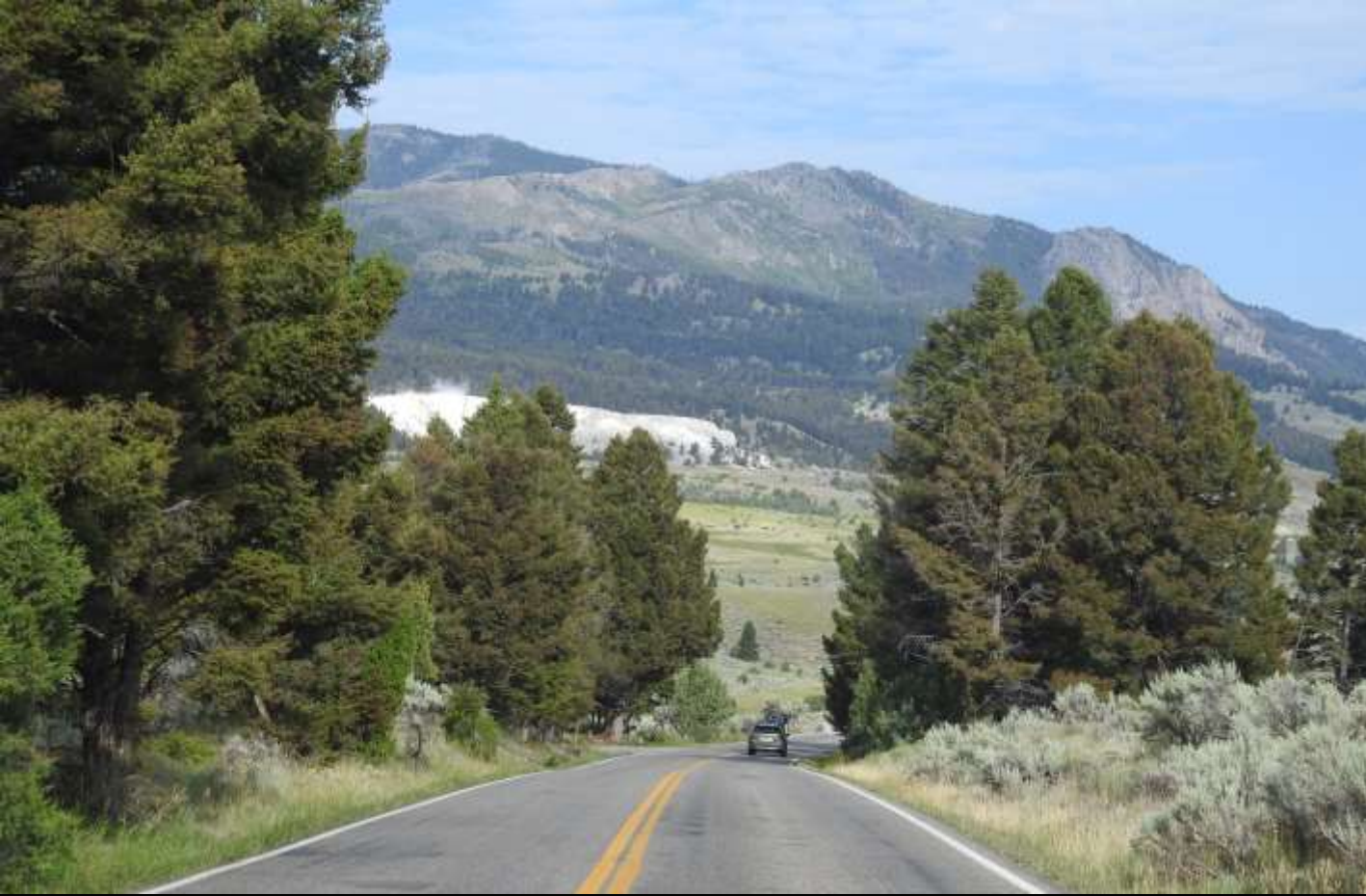
View of Mammoth Hot Springs from above (east) of the Mammoth High Bridge (left), then from on the bridge (right).
